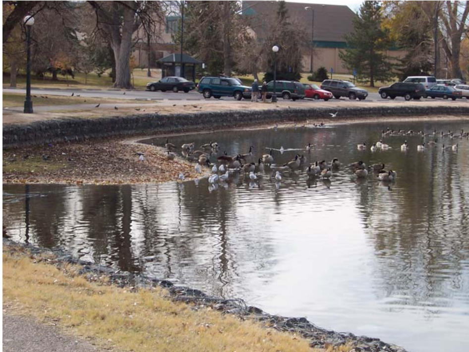
Photo 9 (11/20/2003): Shoreline almost exclusively rock riprap with chicken wire over rock in locations. Bluegrass and trails surround lake.
